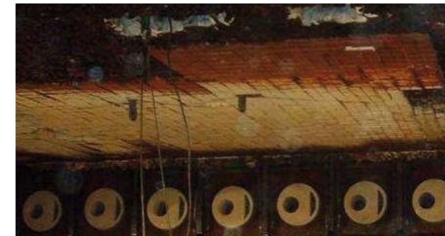
Rebuild of a zone of „normal burners“ to an Ultra Low NOx burner 1610 series
